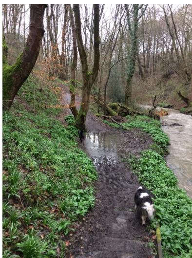
Footpath needing repair in Dean Wood
